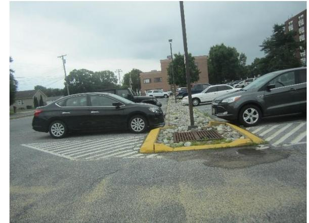
Two sections of parking spaces can be replaced with porous asphalt to capture and infiltrate stormwater runoff from the parking lot. A preliminary soil assessment suggests that the soils have suitable drainage characteristics for green infrastructure.
