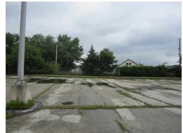
A rain garden can be installed in the turfgrass area near the parking lot entrance west of the building to capture runoff from the impervious parking lot. Porous pavement could be installed in the parking lot in the back toward the northwest of the building to reduce existing pooling and erosion. A preliminary soil assessment suggests that the soils have suitable drainage characteristics for green infrastructure.
