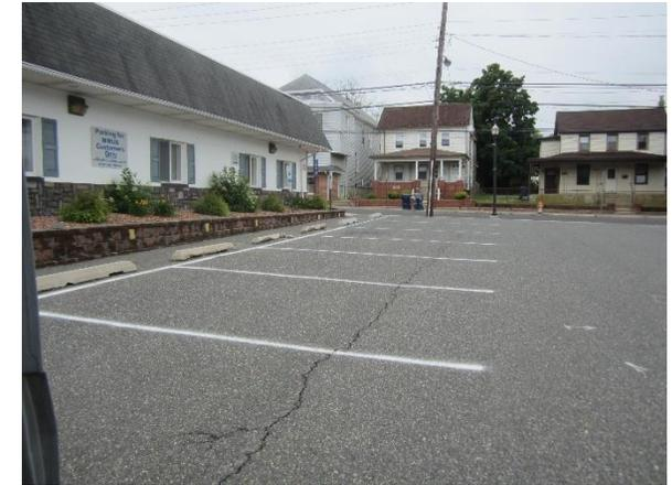
Porous pavement can be installed in the parking spaces near the building to capture stormwater runoff from the roof of the building. A preliminary soil assessment suggests that the soils have suitable drainage characteristics for green infrastructure.
