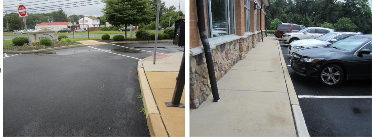
Parking spaces in the parking lot to the southeast of the building can be converted to porous pavement to capture and infiltrate stormwater runoff from the parking lot. A preliminary soil assessment suggests that the soils have suitable drainage characteristics for green infrastructure.
