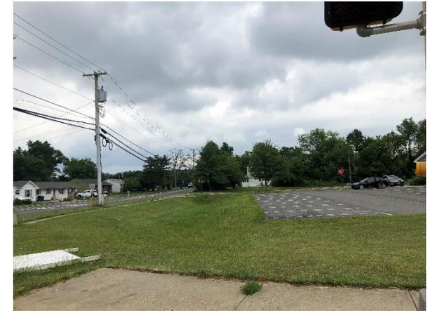
An existing detention basin at the west side of the property can be converted to a rain garden to increase treatment and infiltration of stormwater at the site. Porous pavement can be installed in the parking spaces at the north to capture runoff from the pavement. A preliminary soil assessment suggests that the soils have suitable drainage characteristics for green infrastructure.
